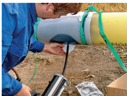
Fig. 4: Filling of the casing sheet
