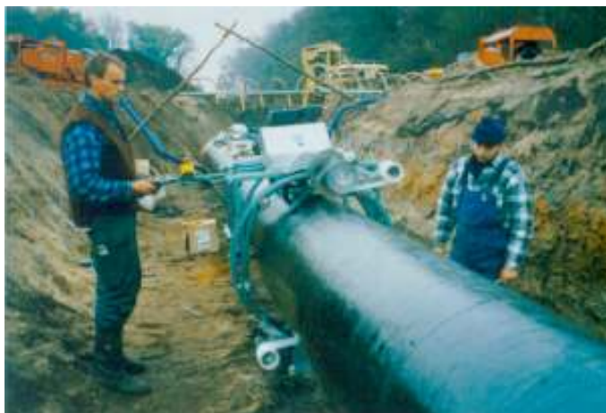
Figure 11: One step application of inner and outer wrap of a DENSOLEN tape system with DENSOMAT 11 wrapping machine
