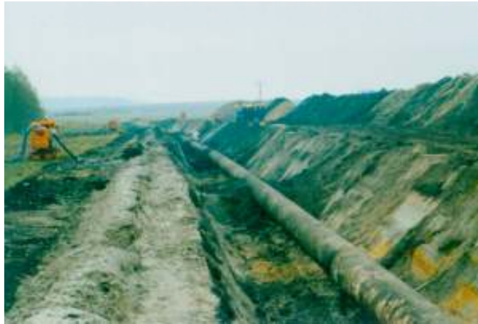
Figure 6: DN 600 bitumen coated pipeline to be rehabilitated while in operation
