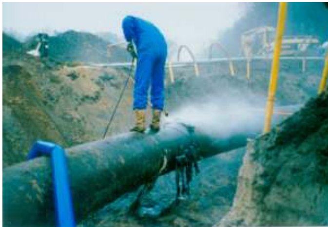
Figure 7: Removal of old coating with high a pressure water jet
