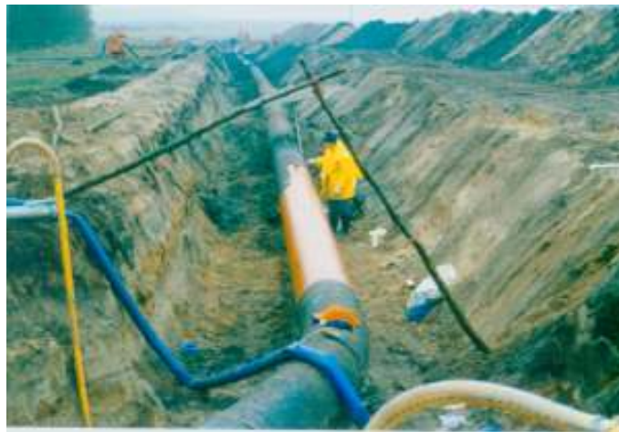
Figure 9: Application of the one component polyurethane primer
