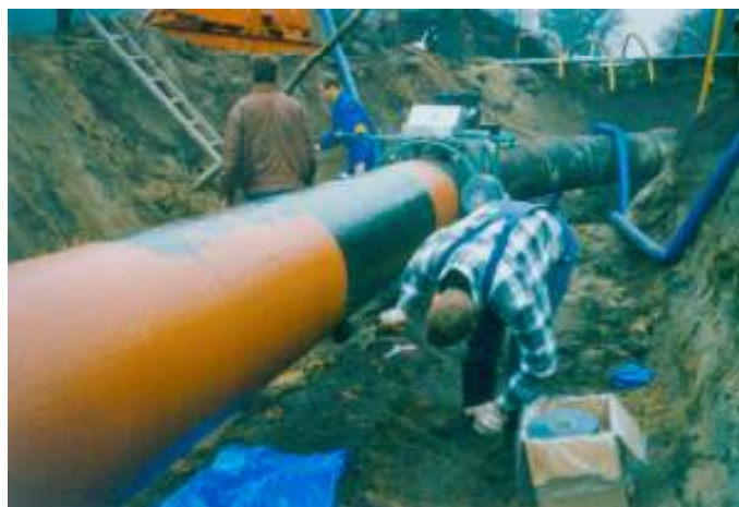
Figure 10: Application of a primer for butyl rubber based tape systems
